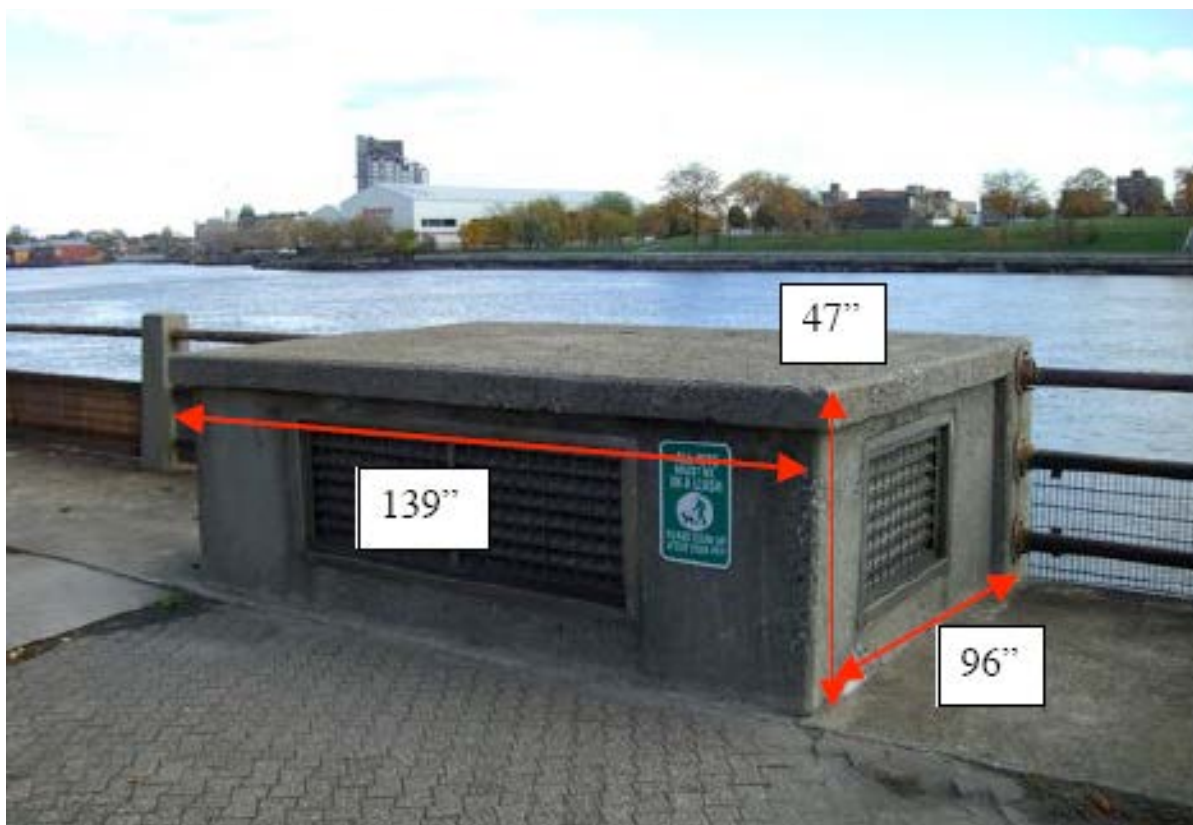
Photo 4.3.8.2-1. Typical Existing Steam Tunnel Vent
